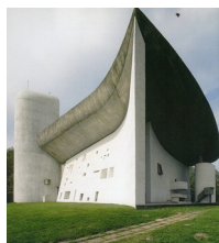
Figure 1: Northeast side of Le Corbusier's chapel at Ronchamp [6].
